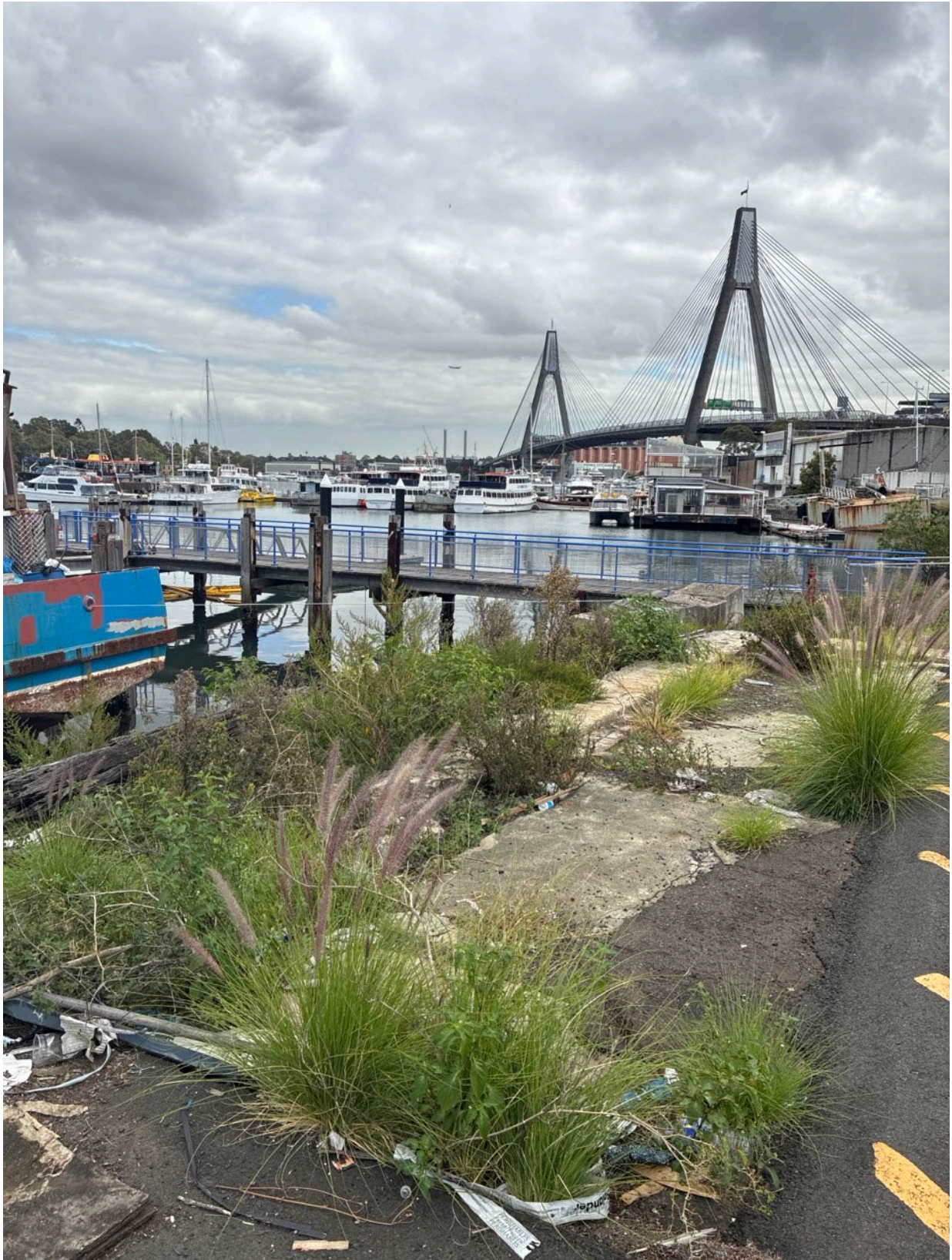
Figure 11: exotic vegetation / weeds which do not represent part of a PCT outside of the demolition area
